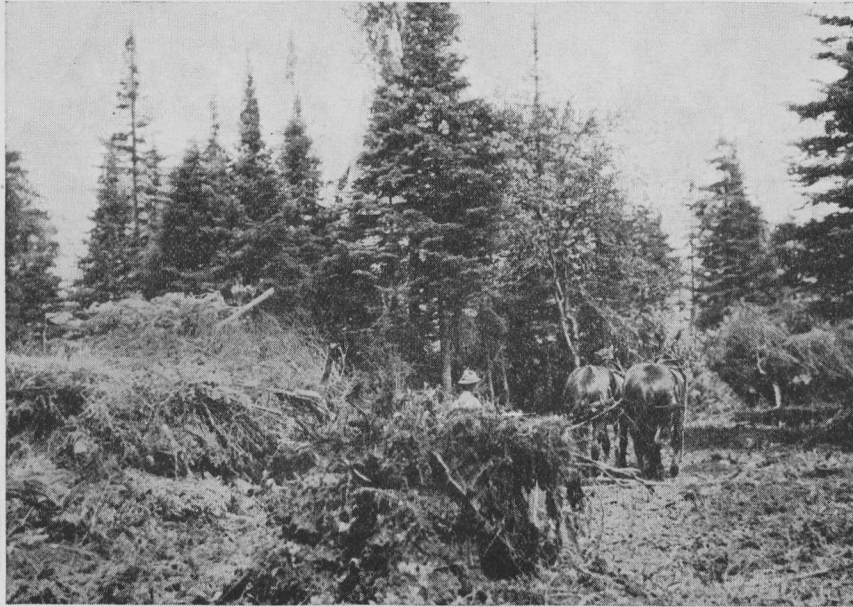
FIG. 5. "OLD BILL" CLEARING THE HORSE BARN SITE, 1913
