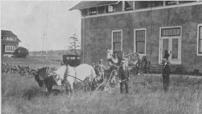
FIG. 8. BREAKING GROUND FOR THE AUDITORIUM, 1929
